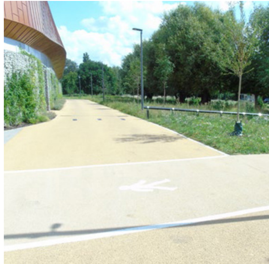
Permeable buff coloured tarmac to main pedestrian and cycle link of the north-south Green spine. Permeable paving chosen to benefit sustainable drainage in line with Dublin City Development plan and national guidelines.
